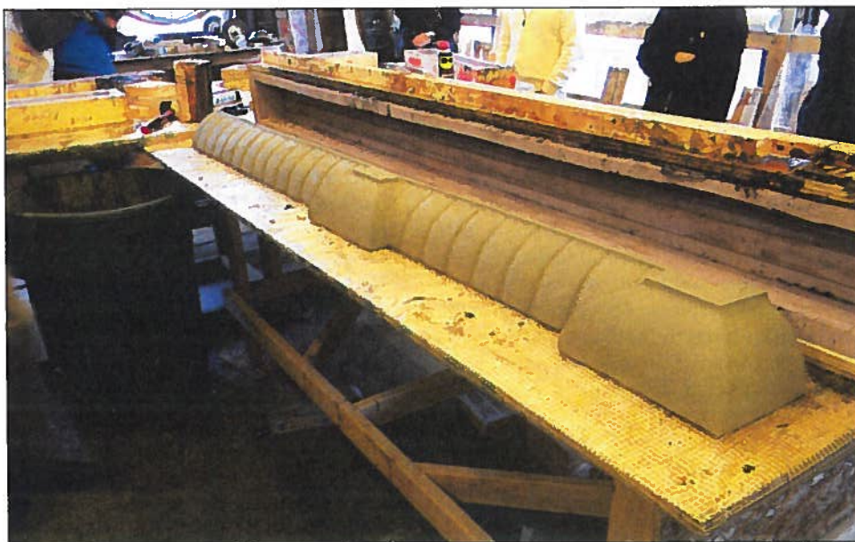
Molds were cast to create composite infill pieces to replicate damaged cast iron detailing around windows on the second, third and fourth floors.
